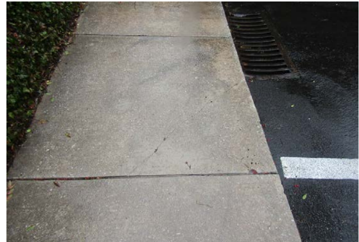
cracked concrete
