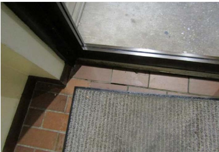
grout damage
