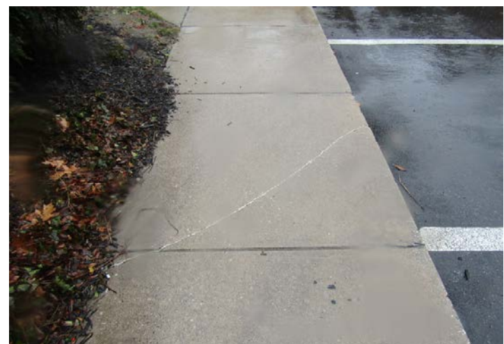
crack in concrete
