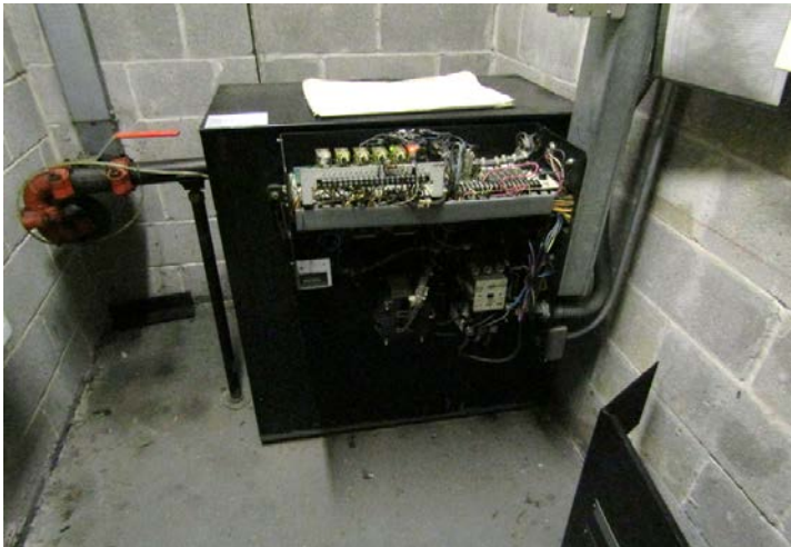
relay logic controls
