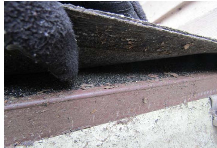
self adhering underlayment at gutter edge
