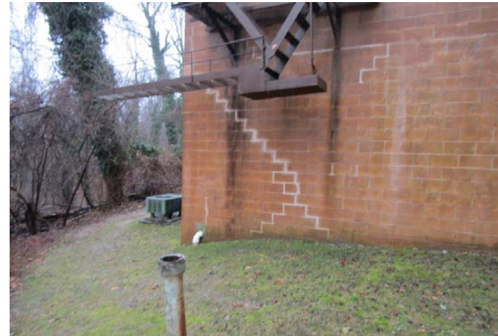
step cracks
