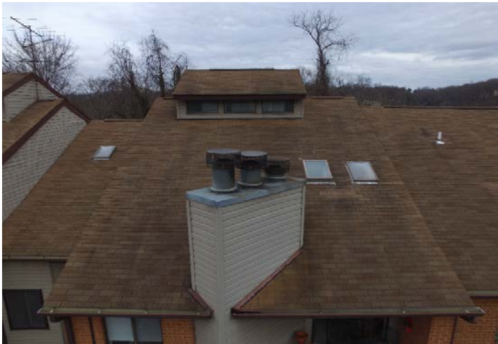
galvanized steel chimney chase cover
