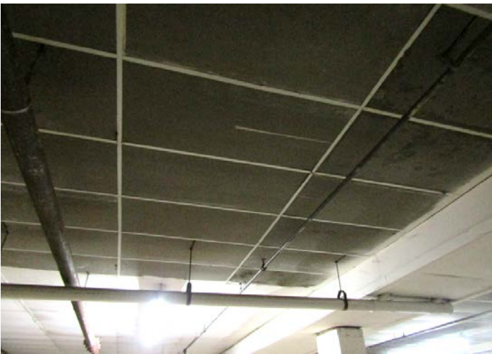
two-foot by four-foot ceiling tile and grid typical of the garages
