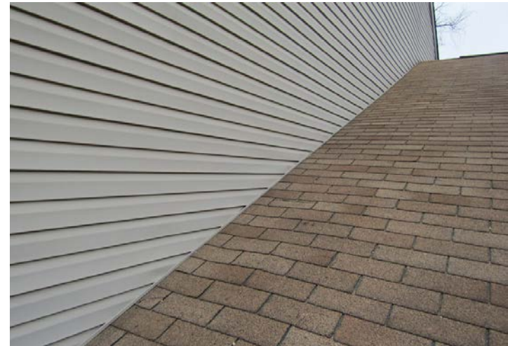
siding in contact with the roof
