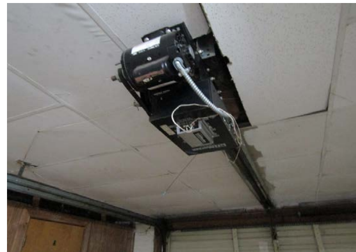
LiftMaster door operator
