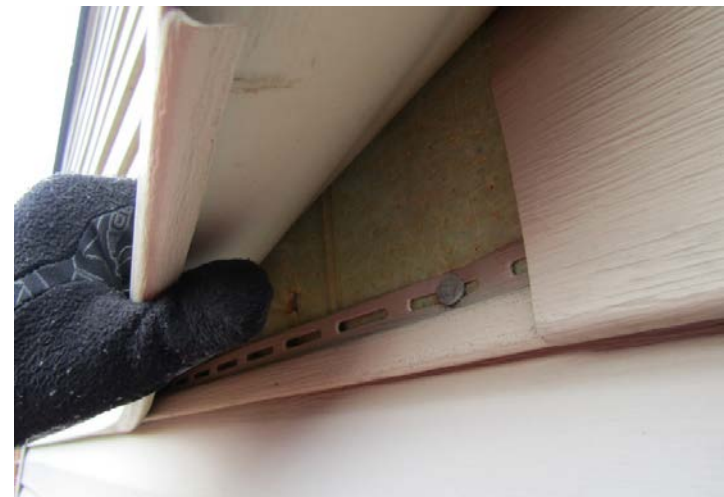
installation missing building paper
