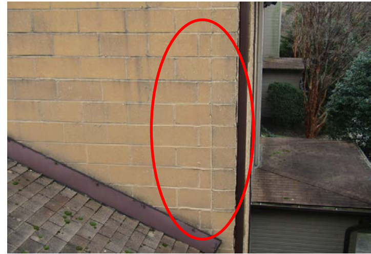
cracks in masonry
