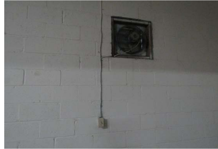
Dayton wall mounted exhaust fan (notice switch in "off" position)
