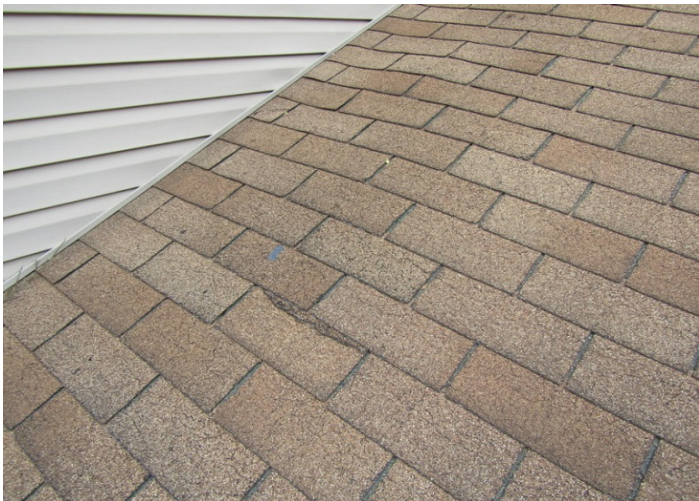
damaged shingles
