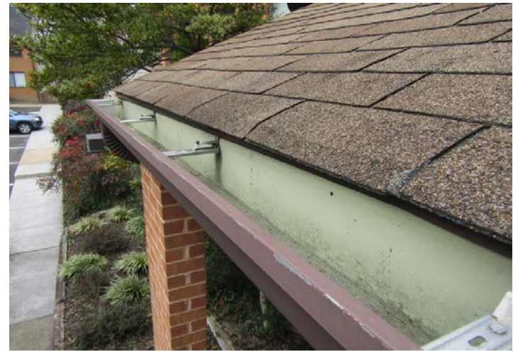
gutters attached with screws
