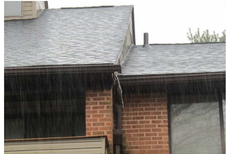
missing downspout at rear of 1704
