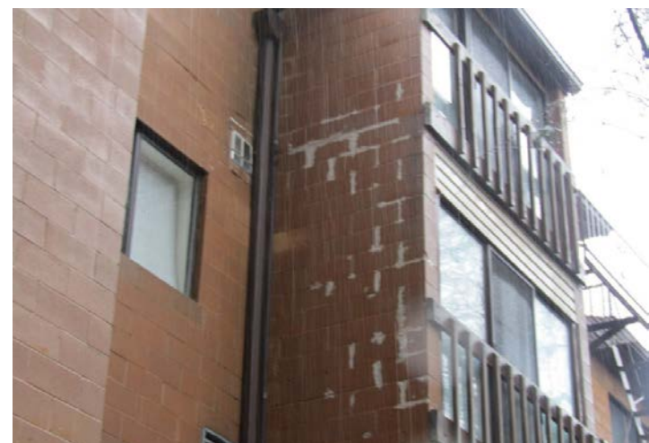
joints repaired with caulk
