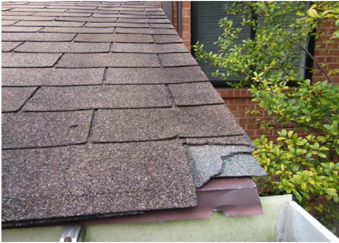
damaged shingles
