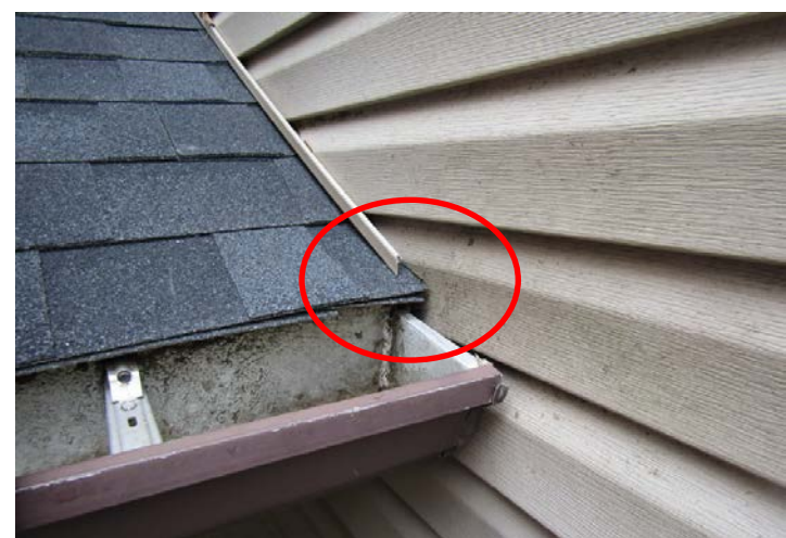
missing kick-out flashing at roof, siding and gutter intersection
