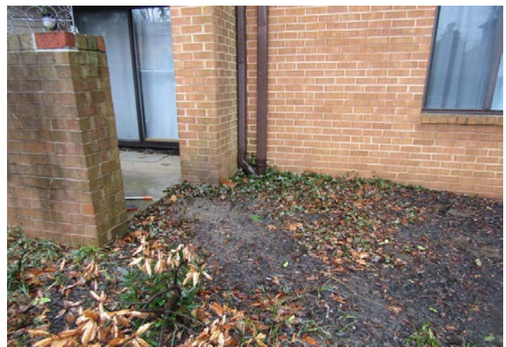
two downspouts at location of leak into garage at 1704
