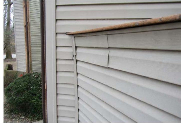
vinyl siding with Dutch lap profile
