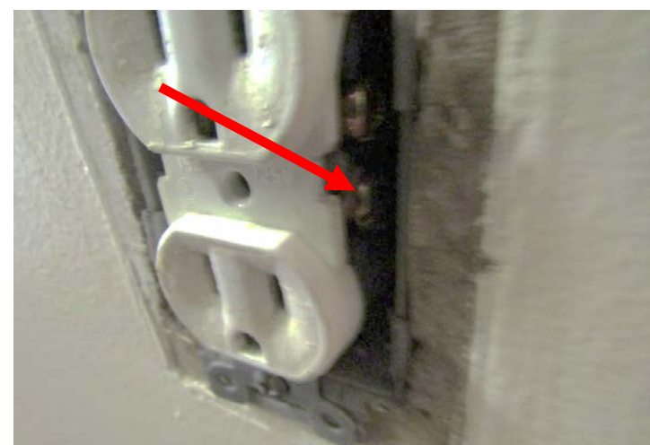
copper wiring
