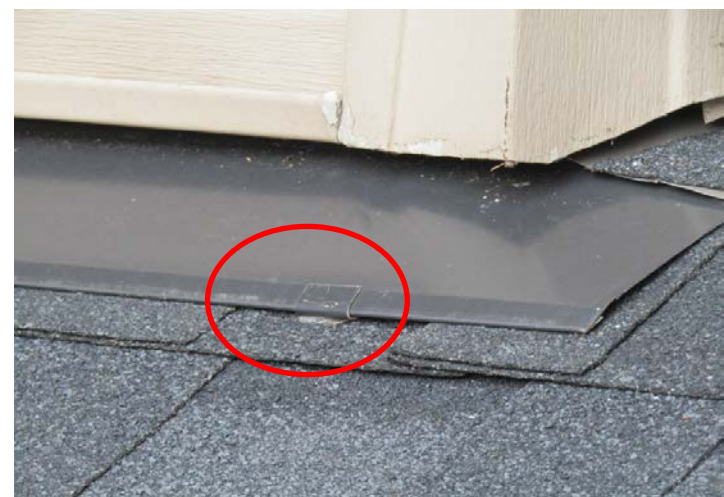
clip holds flashing - very nice detail at new roofs
