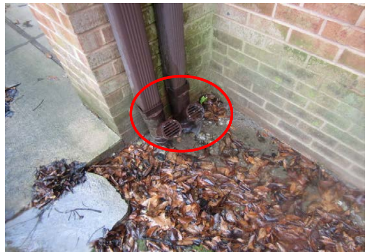
overflowing downspout
