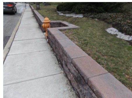
Photo 4 - Modular block retaining wall
